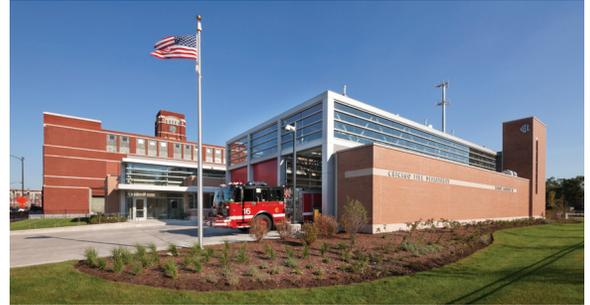
This new 20,063-square-foot Engine Company 16 firehouse features load bearing masonry with exterior brick finish and has been designed to last 100 years, constructed of durable materials that will stand the test of time and the impact of being a 24-hour facility. The facility also includes:
