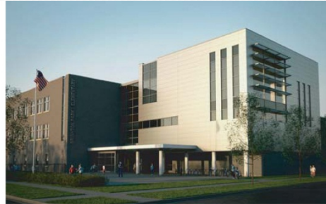
BRIGHTON PARK I ELEMENTARY SCHOOL
