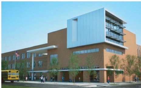
AVONDALE/IRVING PARK AREA ELEMENTARY SCHOOL
