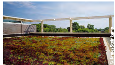
Extensive green roofs include a shallow growing media and require minimum maintenance after plant establishment.
