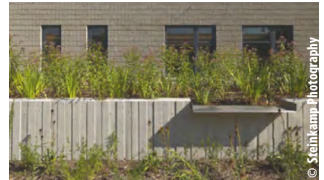
Collected stormwater can be used for irrigation.
