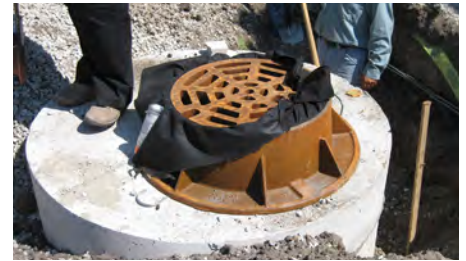
Silt traps control migration of soil particles into the existing sewer system.
