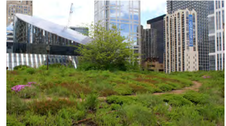
Green roofs mitigate the UHIE and maximize open space.
