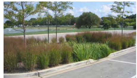
Vegetated filter strips and sedimentation basins filter and temporarily store stormwater on-site and allow sediments to settle.
