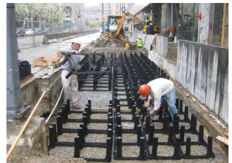
Structural cell systems provide the necessary soil capacity for trees to grow larger.
