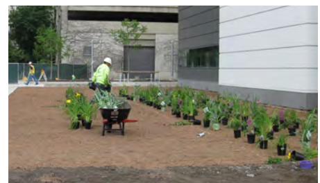
LA shall review plant layout prior to installation.
