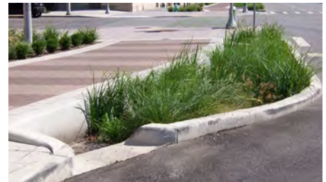
Stormwater management maximizes subsoil infiltration in order to minimize impacts to the City sewer system.
