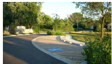
Permeable pavers can be installed as drainage strips in parking stalls.
