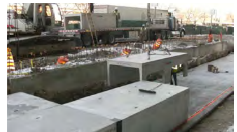
Underground detention tanks temporarily divert collected stormwater from the City sewer lines.
