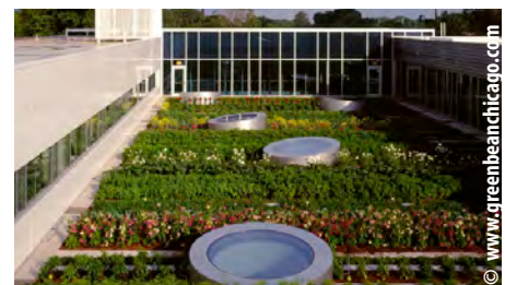
Intensive green roofs include a greater growing media depth and allow for a wide variety of plant options.
