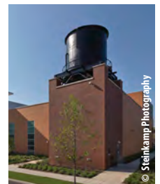
Historic water tanks can be used as cisterns to reduce detention requirements.
