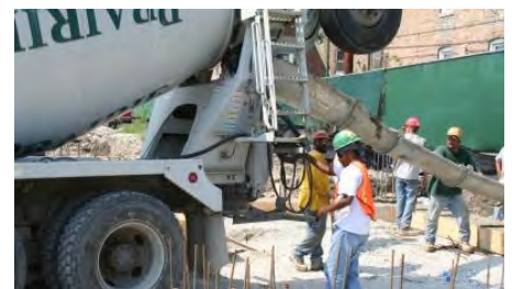
Concrete is a preferred material due to its strength and reflectivity.
