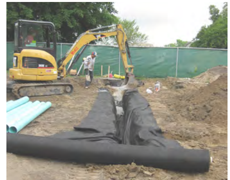
Subsurface drainage may be required to encourage long-term plant health.
