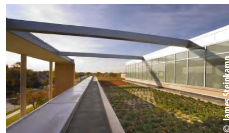
Soil mixes shall be coordinated with the weight the roof is designed to support.
