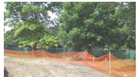
Within the drip line of existing trees, there shall be no grading and the areas shall be protected throughout construction.
