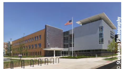
Bike racks shall be located at every major entrance to the facility.
