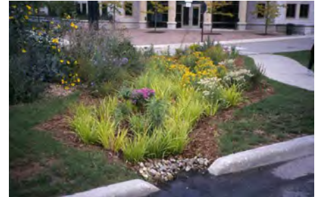
Filtration basins and rain gardens are planted with native plants that slow stormwater runoff from impervious surfaces and allows it to infiltrate into the soil.
