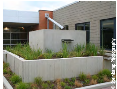
Roofs offer the best source of high-quality stormwater for irrigation.
