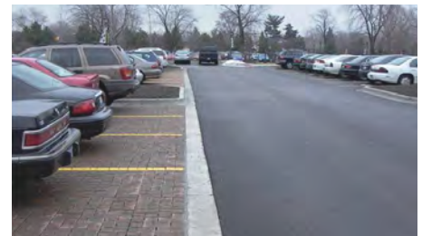
Permeable pavement cleaning is beneficial because it improves the function of water infiltration.
