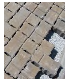
The latest generation of permeable pavers have narrower water intake areas along all sides.
