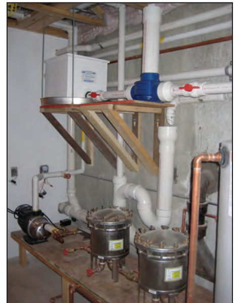
System photograph showing in line filtration from upper left - lint filter, chlorine tablet feeder, greywater tank (to right), 2 micron filters, UV lamp (rear) and pump.
