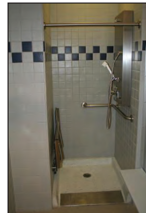
A low-flow shower at the Chicago District 9 Police Station
