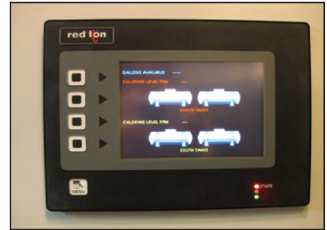
Control System and Monitor
