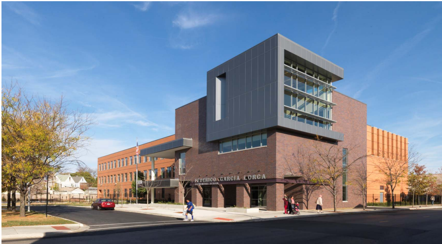
Federico Garcia Lorca Elementary School
