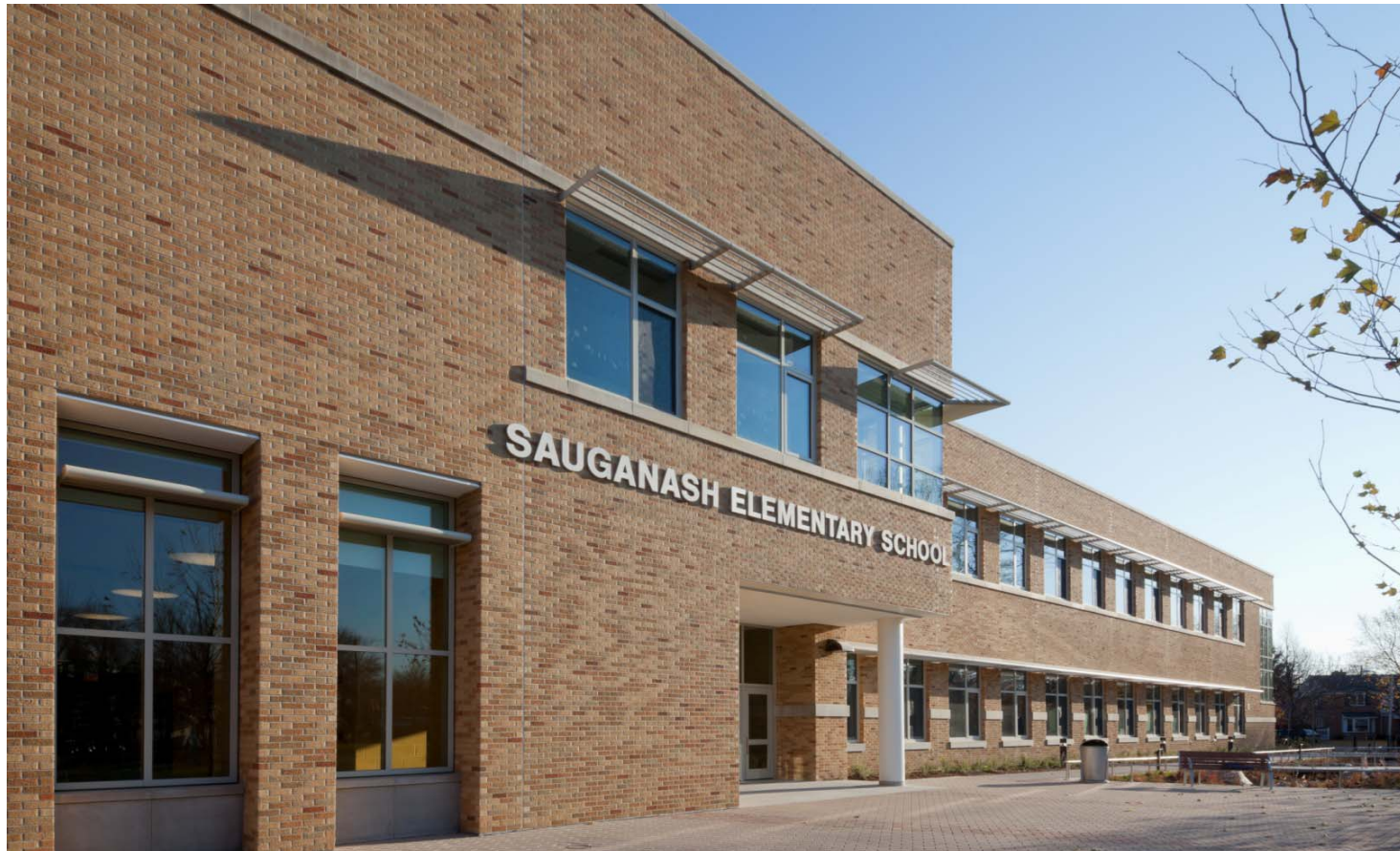
Sauganash Elementary School Addition
