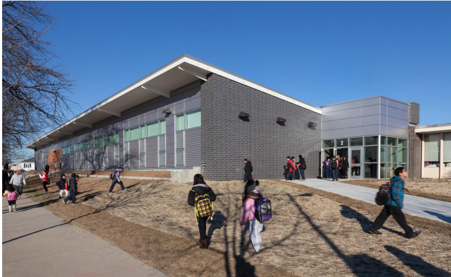
Durkin Elementary School Annex
