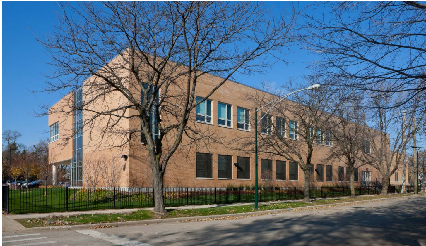
Garvy Elementary School Addition
