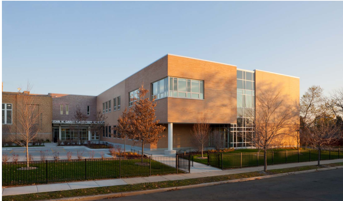
Garvy Elementary School Addition
