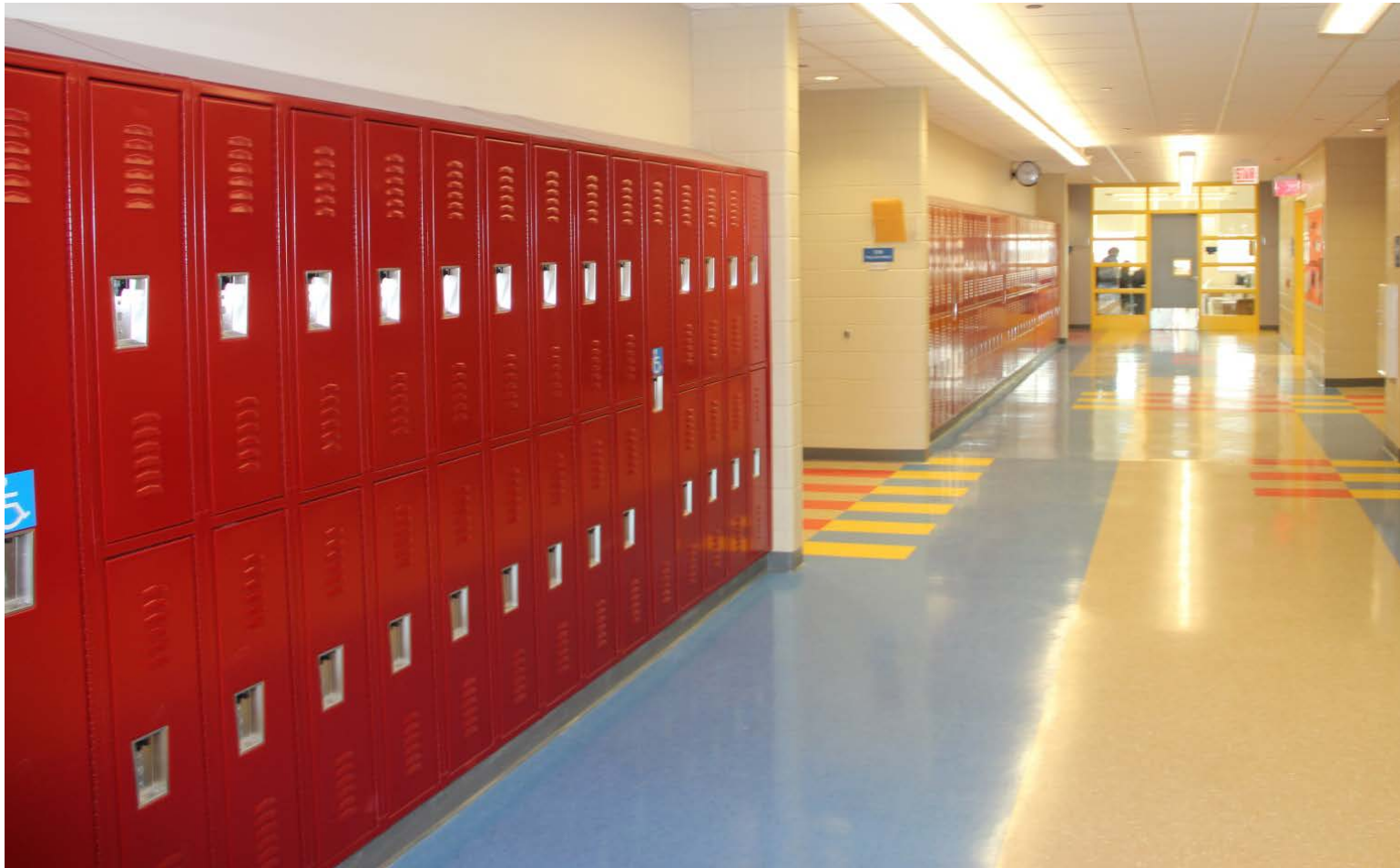
Corridor at Hale Elementary School Annex
