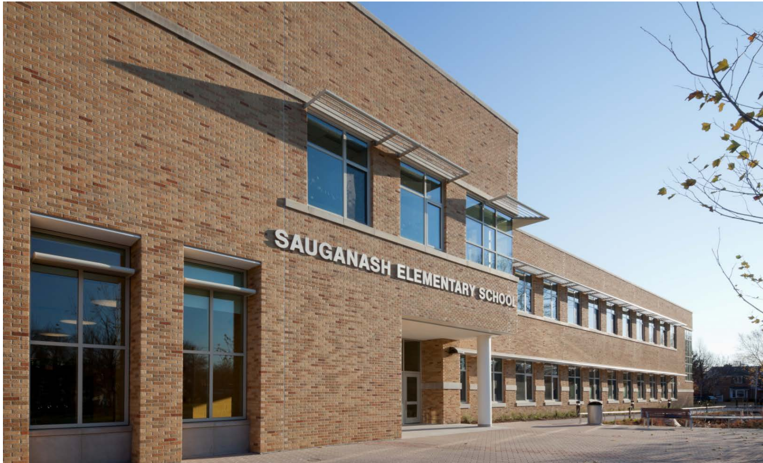
Sauganash Elementary School Addition
