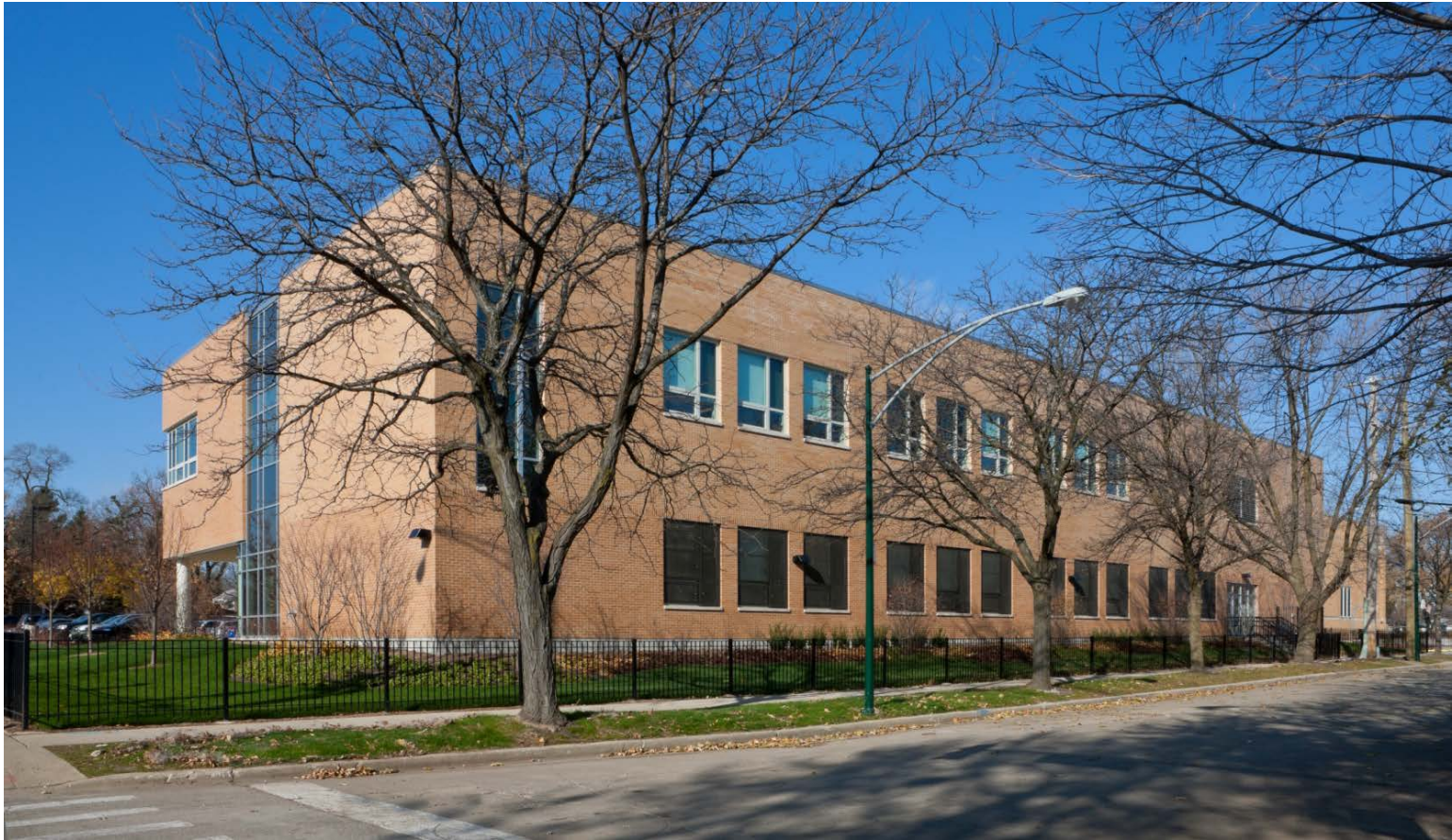
Garvy Elementary School Addition
