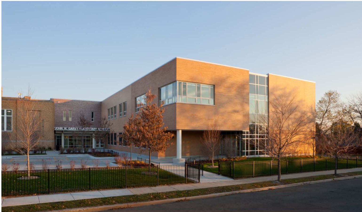
Garvy Elementary School Addition
