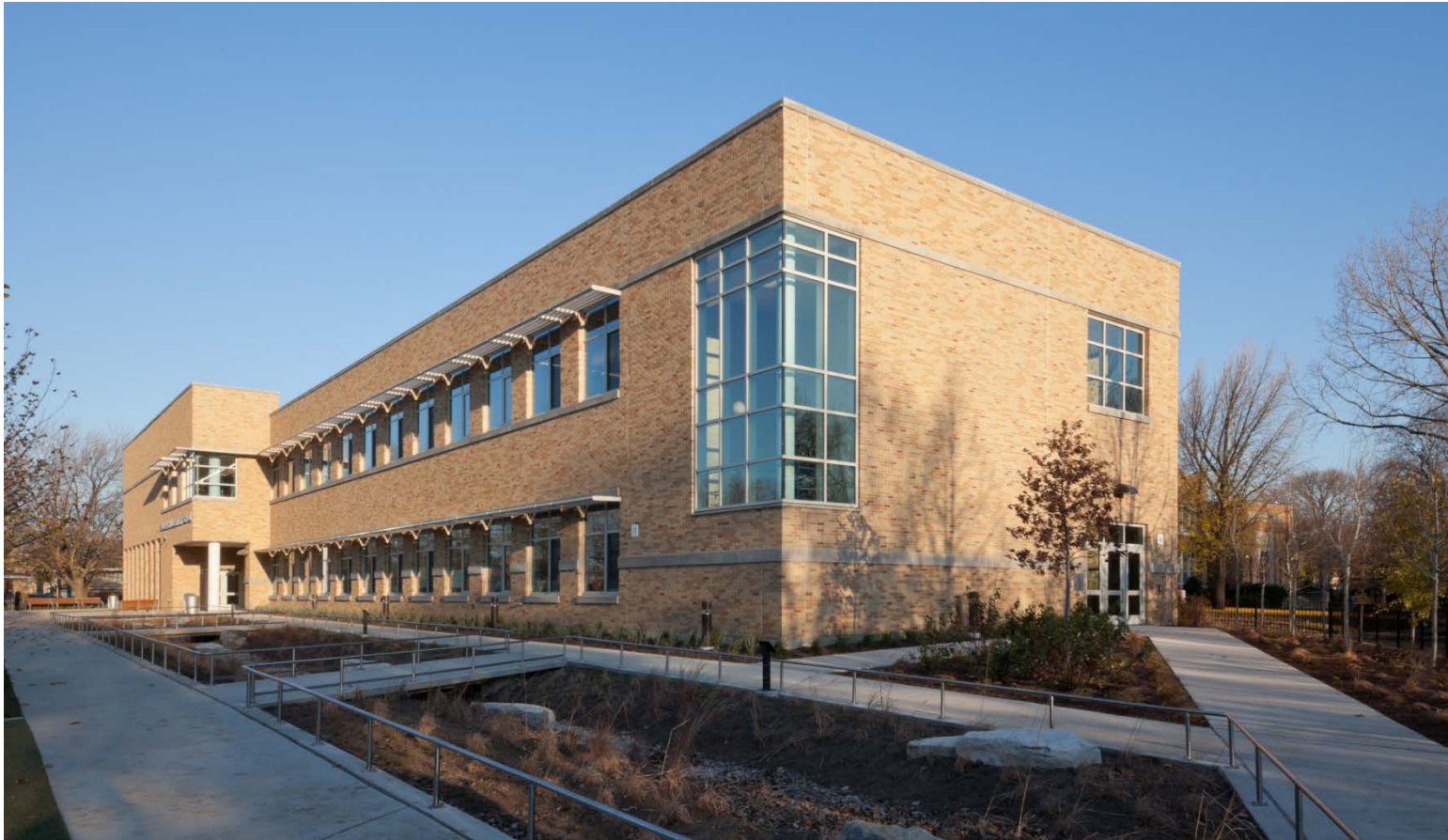
Sauganash Elementary School Addition
