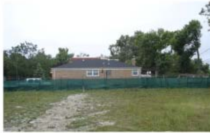
VIEW SOUTHEAST - RESIDENTIAL
