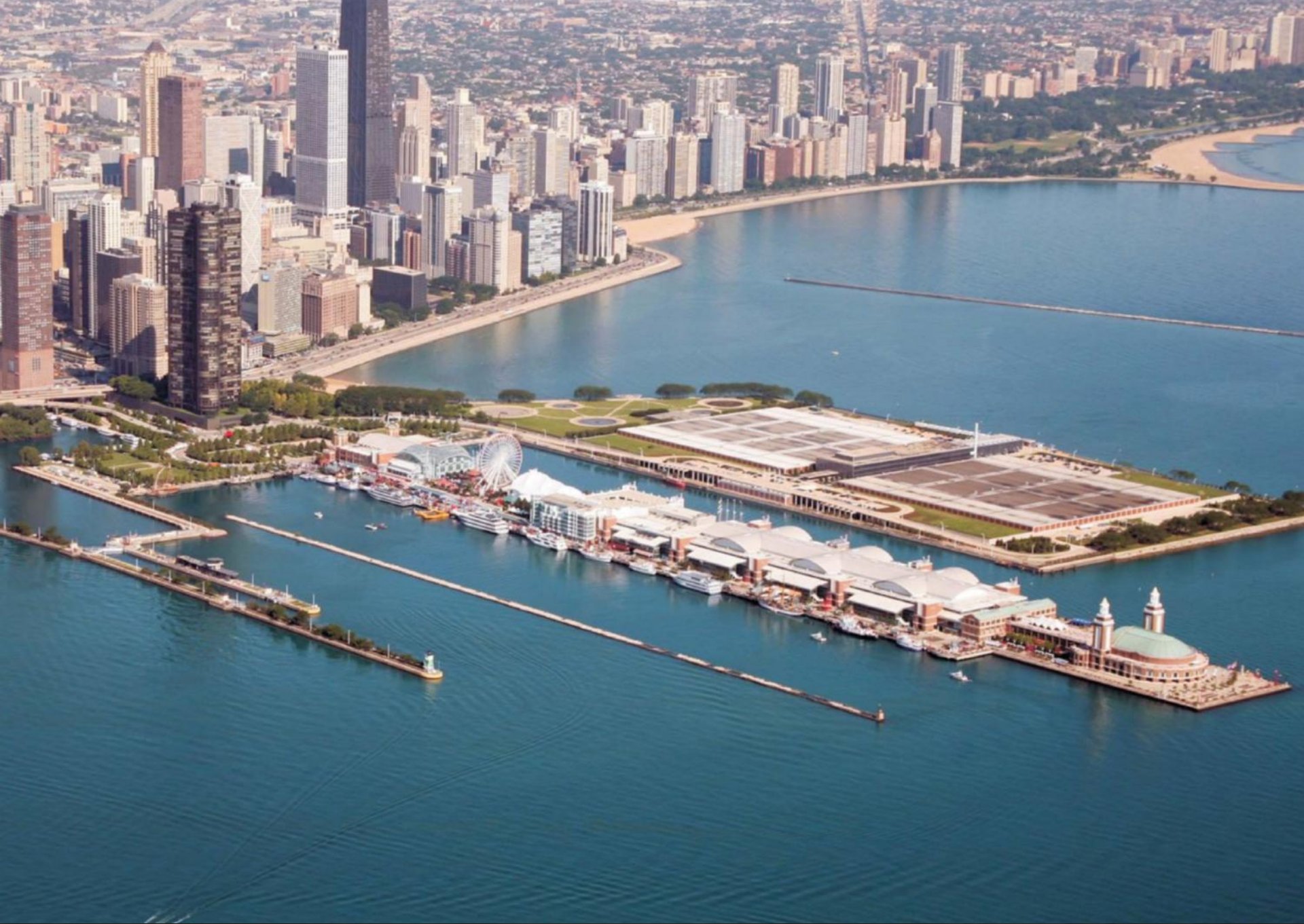
View of Chicago Gateway Harbor Site
