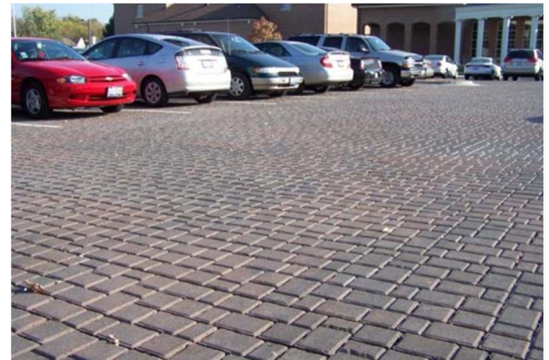
Permeable Pavement Parking Lot Example
