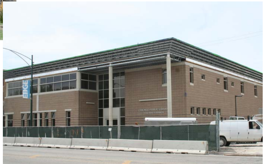
Edgewater Branch: Construction photographs, May 2013
