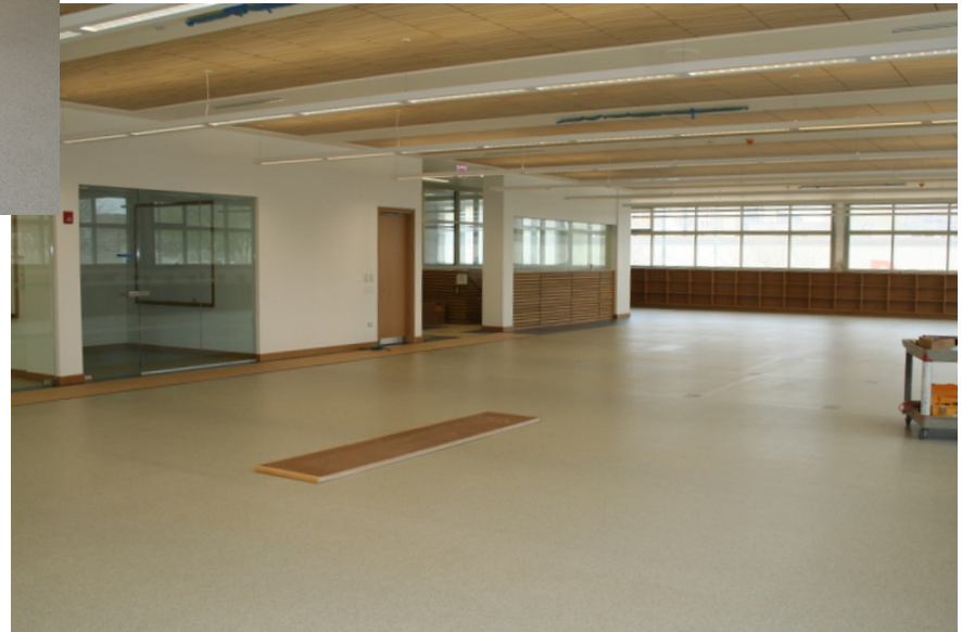
Edgewater Branch: Construction photographs, May 2013
