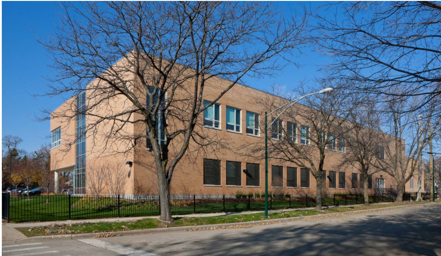
Garvy Elementary School Addition
