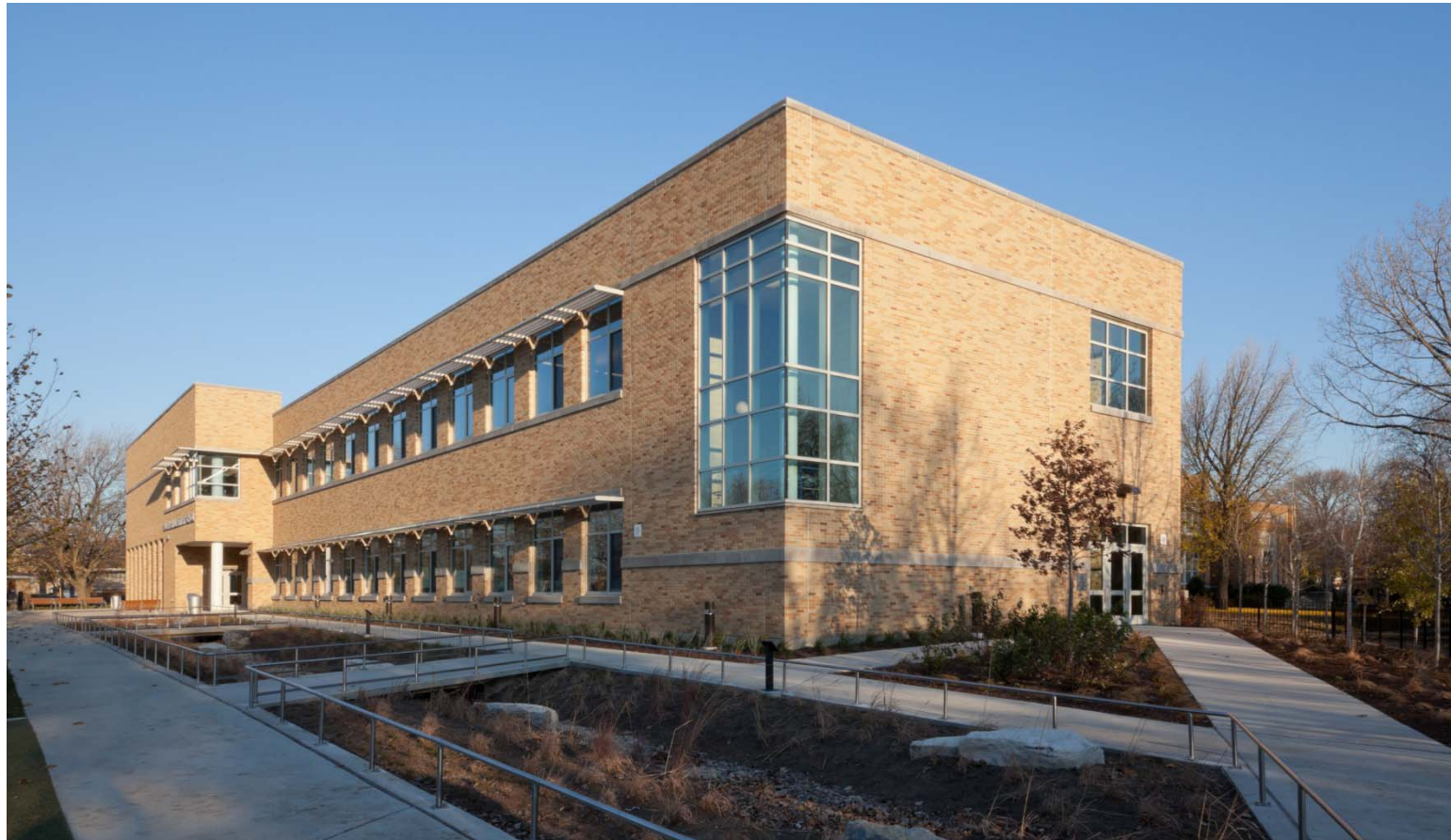
Sauganash Elementary School Addition
