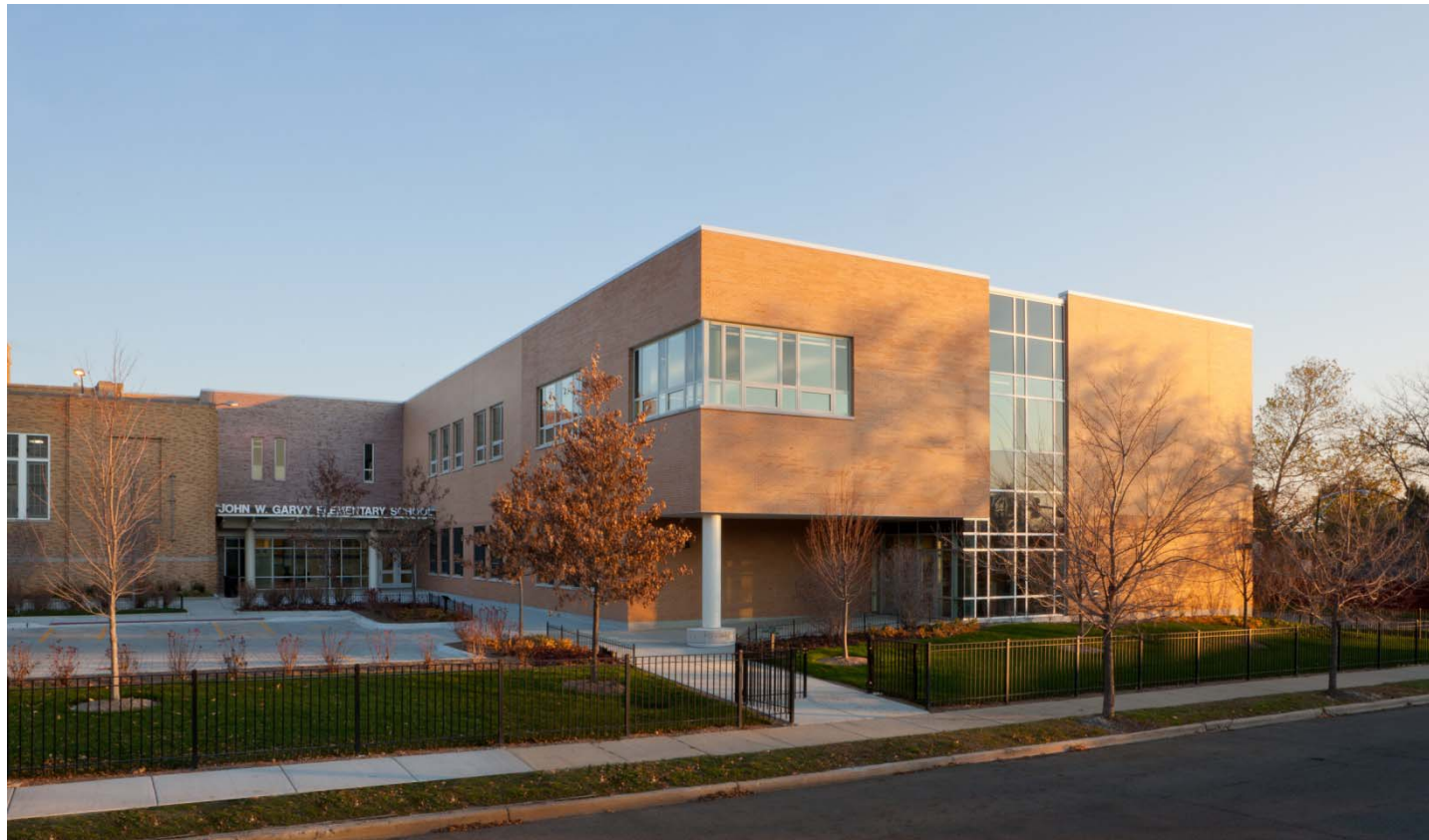
Garvy Elementary School Addition
