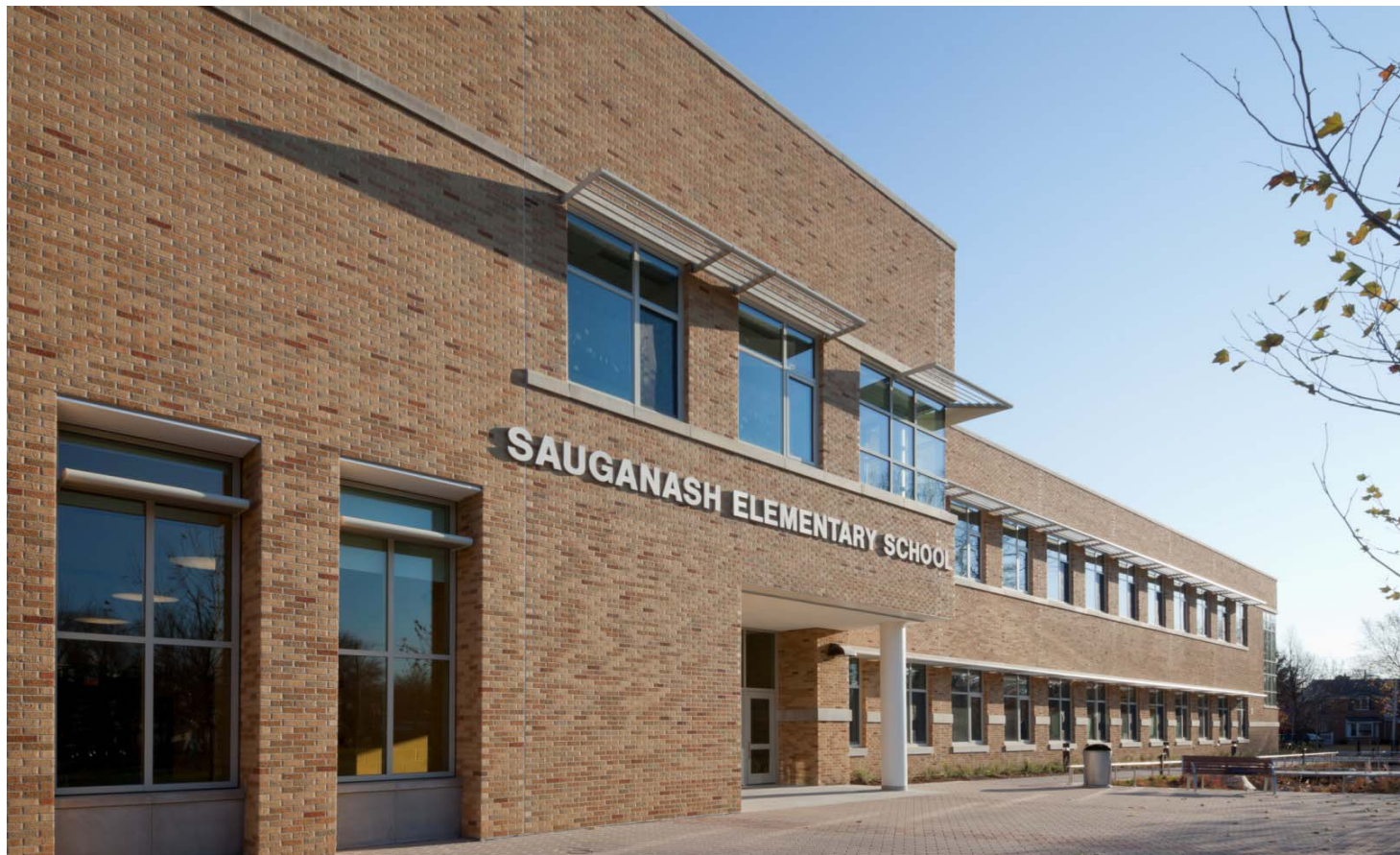
Sauganash Elementary School Addition
