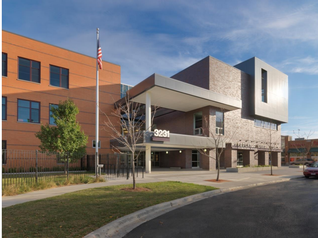
Federico Garcia Lorca Elementary School
